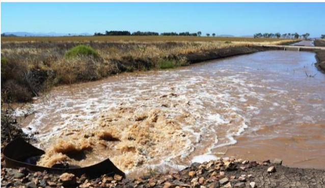
*Figure 3: A diesel pump outside Gunnedah, NSW, diverts water from a nearby river up into an irrigation channel. The water then flows down the channel and is used to flood-irrigate the surrounding fields. Excess water from the channel is stored in an open reservoir.*
