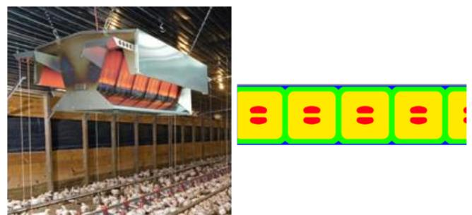
Figure 5: Shenandoah Generation 2 Quad-Glow radiant gas heater and its heating pattern (at floor level) (Shenandoah Corp., n.d.).
