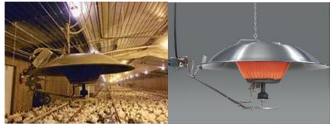
Figure 3: Radiant gas heaters, or ‘brooders’. From (Owens & Ray, 2013) and (GSI Inc.).
