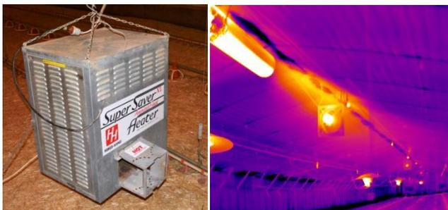
Figure 2: Indoor forced-air gas heater (left) and an infra-red image of a perforated heat distribution duct from an external gas heater with additional back-up radiative heaters (right) (University of Georgia, 2009).
