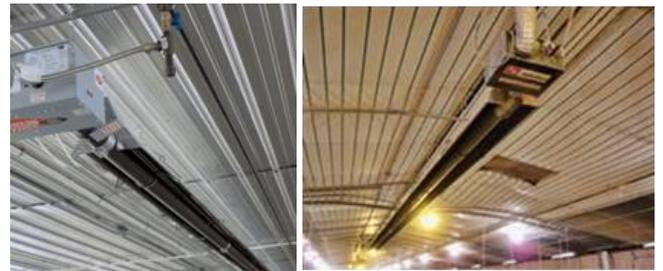
Figure 4: Figure Examples of radiant tube heating; note that the combustion chamber (burner or firebox) is the box at the end. From (GSI Inc.) and (Owens & Ray, 2013).
