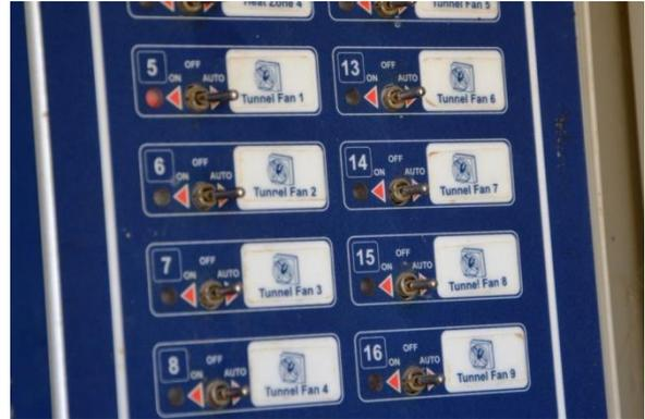
*Figure 2: Controls for ventilation fans in a poultry shed.*
