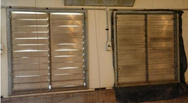
*Figure 1: These ventilation fans have shutters to block air flow when they aren't running. You can see light (and air) streaming through the shutter on the left, while the shutter on the right has been sealed to control air flow. Shed doors and other passive ventilation points also allow unregulated air into a building and can result in significant avoidable energy usage (Source: NSW Farmers).*
