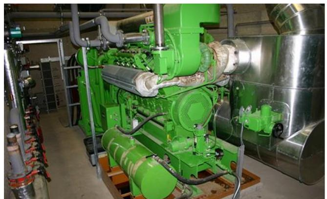
Figure 4: A typical industrial scale gasifier, gas fired engine and generator that can power a whole farm. Massive energy cost savings but big capital upfront as well as ongoing maintenance
