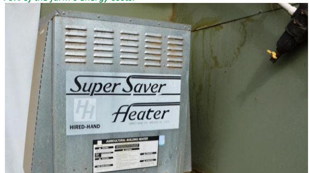
Figure 4: LPG-powered heaters will need conversion to biogas if the business case for Stratheden Glen's waste-to-energy opportunity is realised. These heaters use 50% of the farm's energy use and account for 70% of the farm's energy costs.
