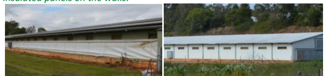
Figure 5: Left: One of Will's older sheds, with a polymer curtain providing part of the lateral building envelope. Right: One of Will's newer sheds, with insulated panels on the walls.
